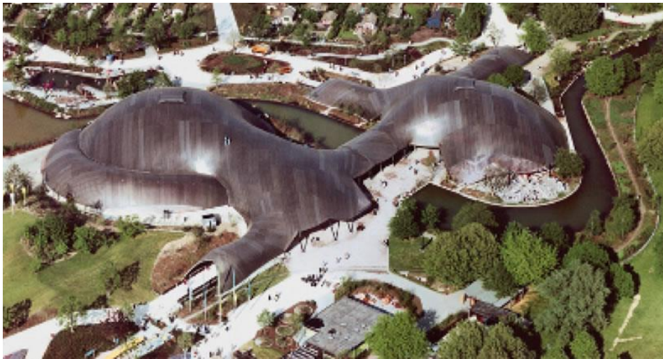
Fig. 221. Centro Multifuncional de Mannheim. Fuente: https://www.designboom.com/architecture/frei-otto-a-life-of-research-construction-and-inspiration-detail-book-report-06-02-2015/ .jpeg
