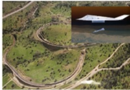
Figure 2. Railway section to be destroyed
