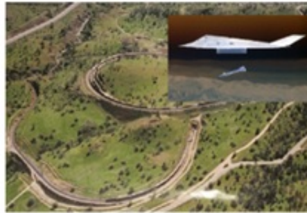
Figure 2. Railway section to be destroyed
